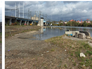
Tidal Flooding in Northeast of Site
