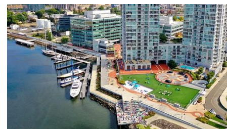
1.0g — Harbor Pt North Marina, Stamford CT
