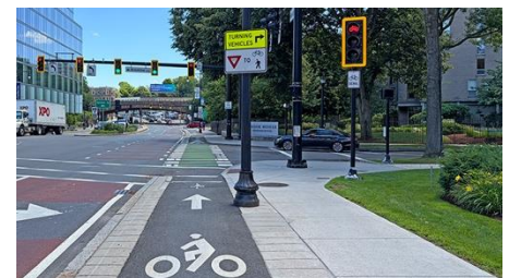
2.1f — Pedestrian-bike sharing path, Washington St at Brookline Ave, Brookline MA
