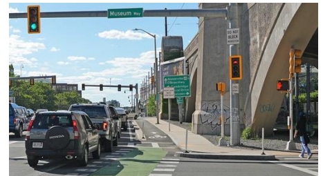
2.1d — Pedestrian-bike sharing sidewalk, Charles River Dam Rd at Museum Way, Cambridge MA
