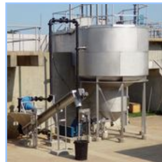
Example of Finished Install
