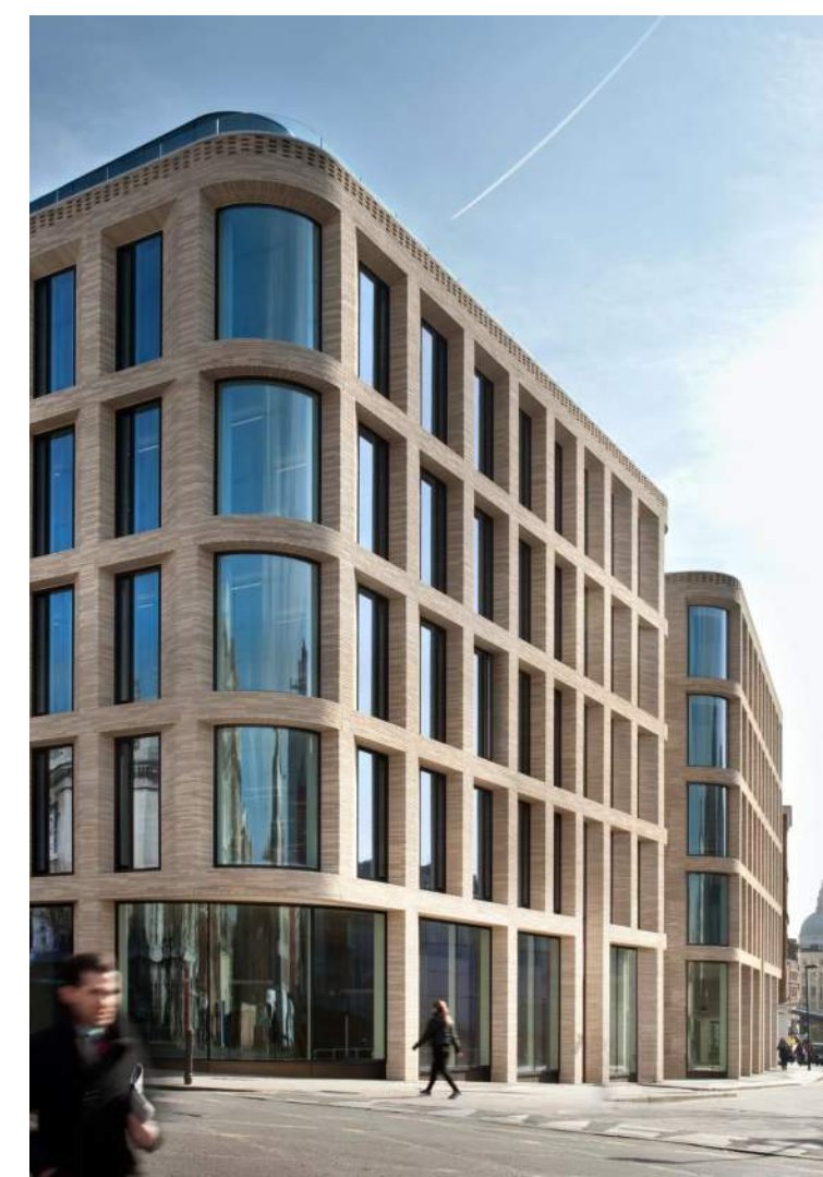
MODERN PRECEDENT TURNMILL BUILDING LONDON
