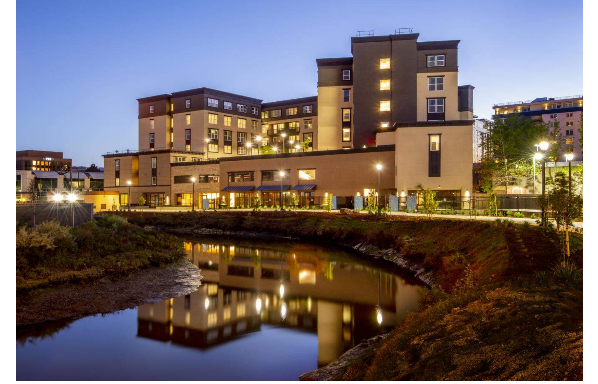
Arroyo Green – completed in 2021
