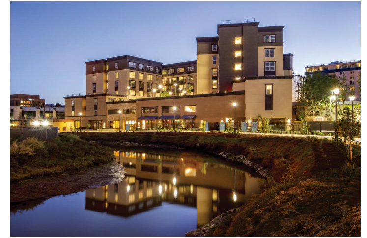
Arroyo Green – completed in 2021
