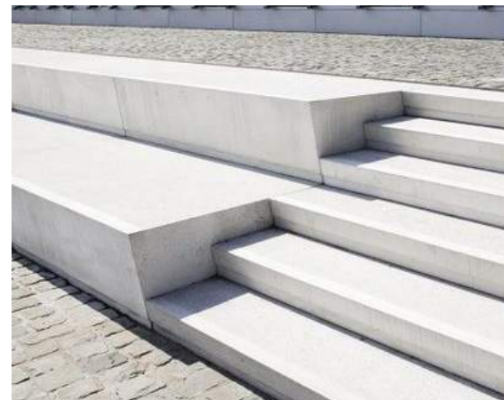
Precast Concrete Seat Wall
