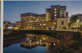
Arroyo Green - completed in 2021
